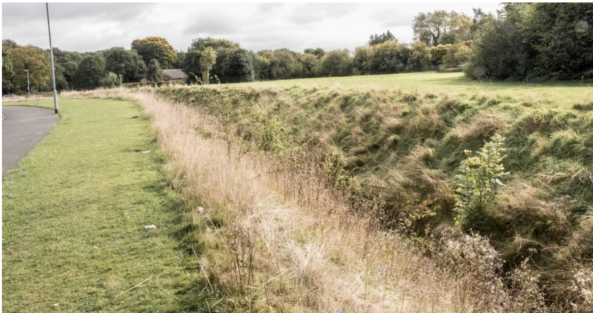
Figure 8: The grassed area pictured to the right of the channel (true LB) is potentially space available for re-meandering and floodplain re-connection opportunities.
