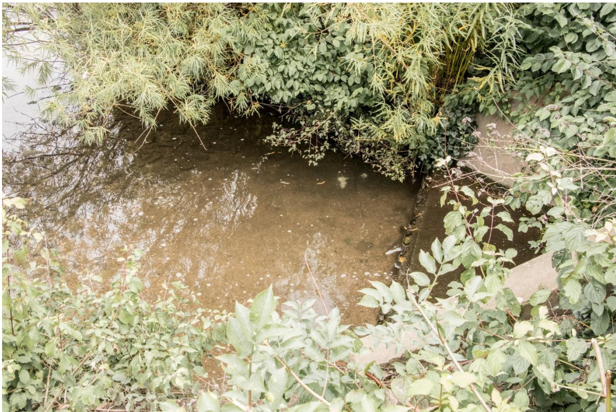
Figure 9: Lake inlet receiving the River Penk as it emerges from culverting.
