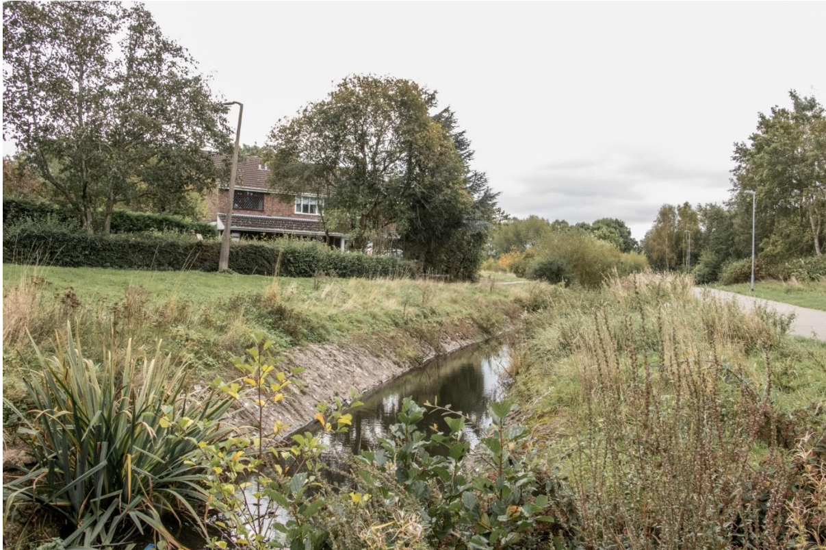
Figure 12: More open section of channel - which still draws complaints requesting vegetation removal.
